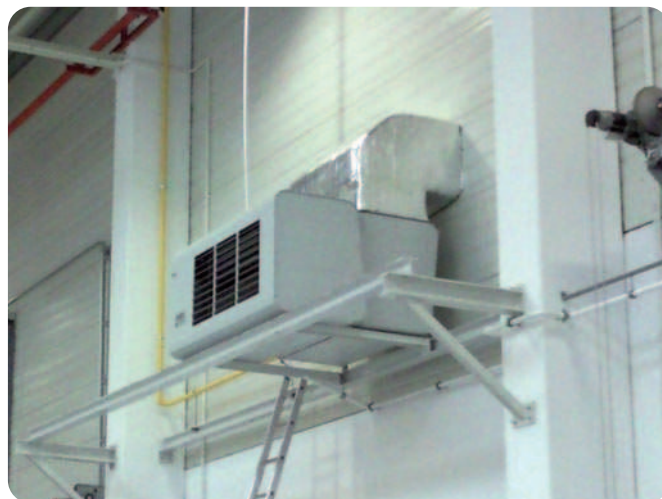
EXTERNAL AIR INTAKE
