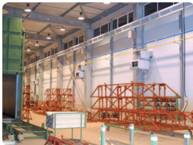
INTERNAL-EXTERNAL RECIRCULATED AIR WITH AIRLOCK
