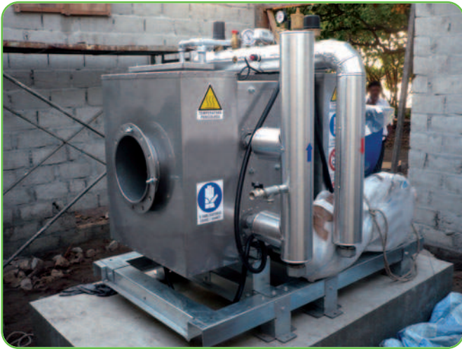
ROME - Biomass 340 kW bigeneration HOT WATER + CHILLED WATER
