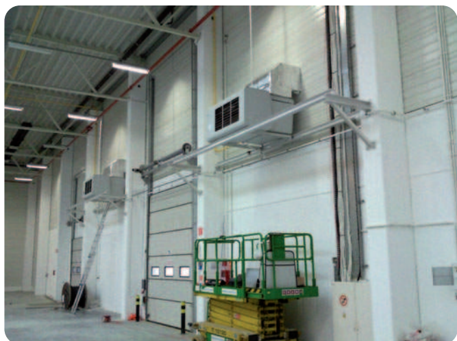
INTAKE OF ONLY EXTERNAL AIR
